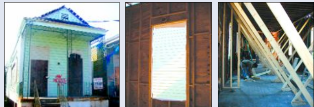
5124 Dauphine St. (left) and 717 Deslonde St. in Holy Cross
